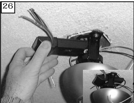
26 Install remote receiver by sliding into opening in the Mounting bracket. Make sure that the dip switches on the Transmitter and the Receiver are set to the same position. See Fig 57 for remote operation
